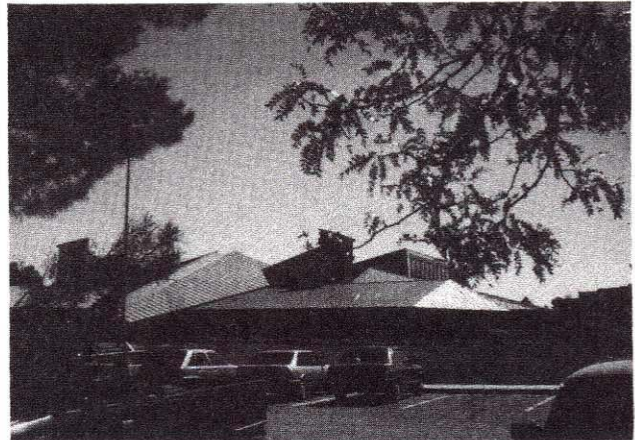
The pool at the South Boulder Recreation Center is a pivotal part of the city's recreation programs, making renovation of the structure on a tight time-frame a high priority for city officials.
