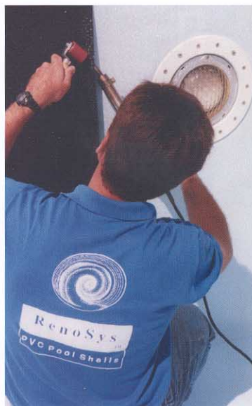
Hot air thermal fusion welding bonds the liner. Compression flanges secure it at penetrations.
