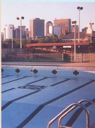
The RenoSys system upholsters the pool with a durable watertight easy to clean membrane.
